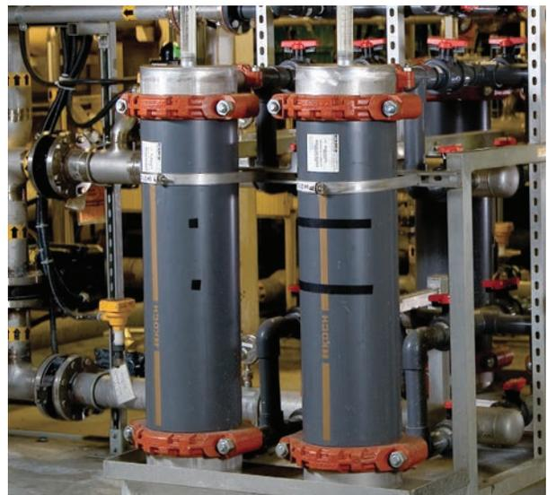
“The decision was not difficult, because no other membrane vendor offered a 10-inch solution,” said Wright. “The 10-inch membranes gave us the capacity we needed with far fewer membranes and much less equipment, compared to systems with 8-inch modules. Our two new KPAK® PLUS systems now sit on the same footprint as the ones they replaced, and yet the new systems provide four times the UF capacity.”
