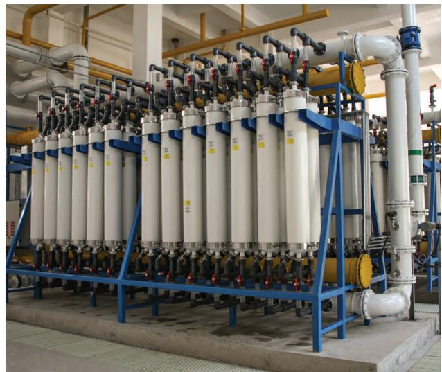
“We analyzed membranes from three vendors and we selected the KSS membranes because our analysis determined that their UF membranes were especially effective at handling the colloidal silica in boiler feed water,” Mr. Srinivasan said.
